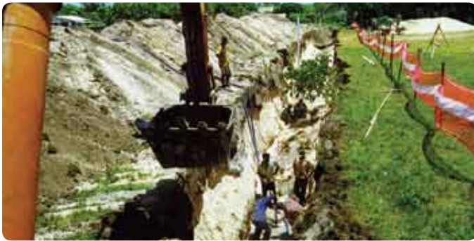
Digging of infiltration galleries.
