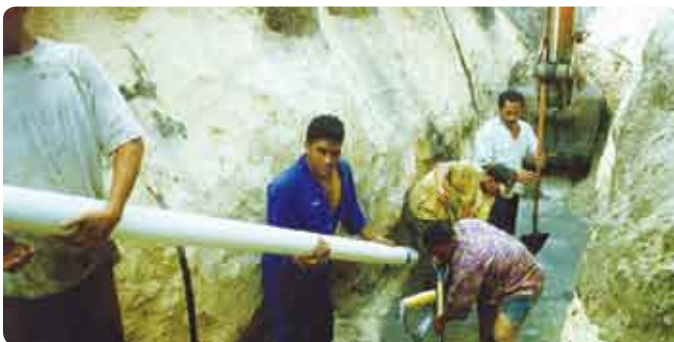
Installation of infiltration gallery floor and pipe work.
